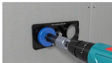
Optional: Mill out additional drill holes with the drilling template (P102-74) to save time and ensure accurate measurements.
