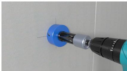
Mark the first box and drill a 74 mm drill hole.
