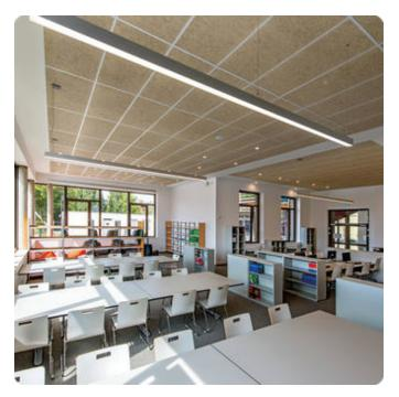
Matching luminaire's surface colour. High-power current. 7863lm. 70W. 7kg. Binning initial <= MacAdam 3. IP20. Protection class I. CE, UKCA marking. Prüfzeichen: ENEC. IK02. 220-240V. 50-60 Hz. RG0 (EN62471). Luminous flux reduction up to 0,4%/1.000 operating hours. Nominal failure rate: 0,2%/1.000 operating hours. L80B10 (tq 25°C) = 50.000h. 5 years warranty. Manufacturer: Lightnet GmbH, ISO 9001:2015 and 50001:2018 certified.
