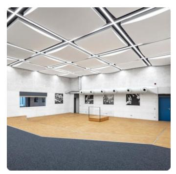
current. 820Im. 9W. 1,8kg. Binning initial <= MacAdam 3. IP20. Protection class I. CE, UKCA marking. Prüfzeichen: ENEC. IK02. 220-240V. 50-60 Hz. RG0 (EN62471). Luminous flux reduction up to 0,2%/1.000 operating hours. Nominal failure rate: 0,2%/1.000 operating hours. L90B10 (tq 25°C) = 50.000h. 5 years warranty. Manufacturer: Lightnet GmbH, ISO 9001:2015 and 50001:2018 certified.
