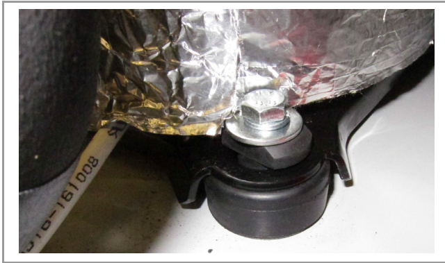
Fig. 3.3:Vibration base for compressor
