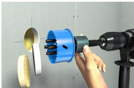
Hold the aluminum sleeve and allow the drill core to be ejected by turning the drill to the left.
